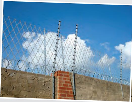
Domestic Fence, Kyalami (SA)
