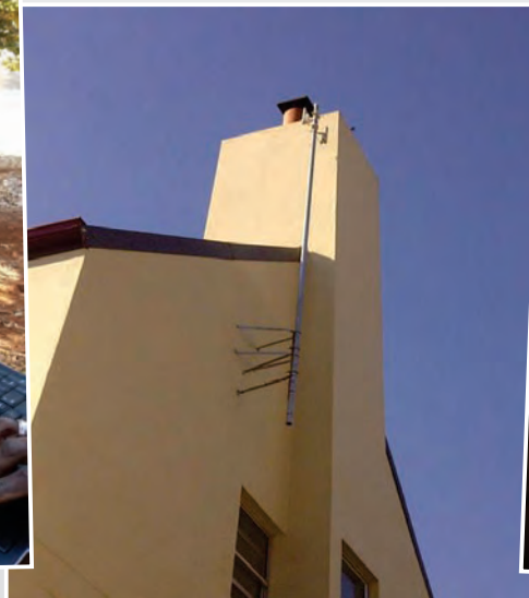
Wireless Transceiver at Control Room
