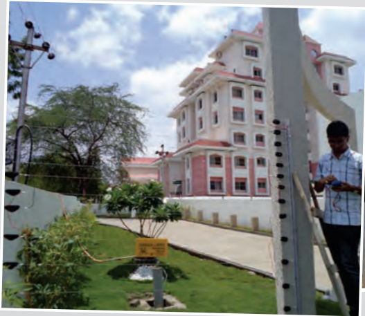
Security Fence Installation, India
