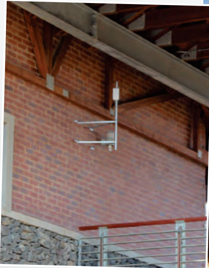
Wireless Transceiver Installation
